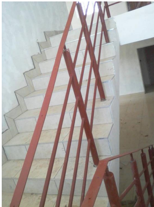
Figure 23 fabrication and installation of Mild Steel Handrails
