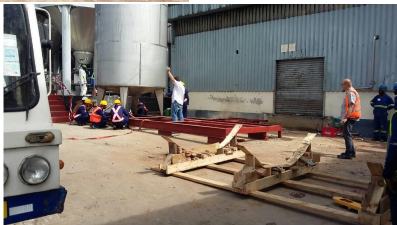
Figure 25 fabrication and Installation of Steel storage tanks at Carlsberg
