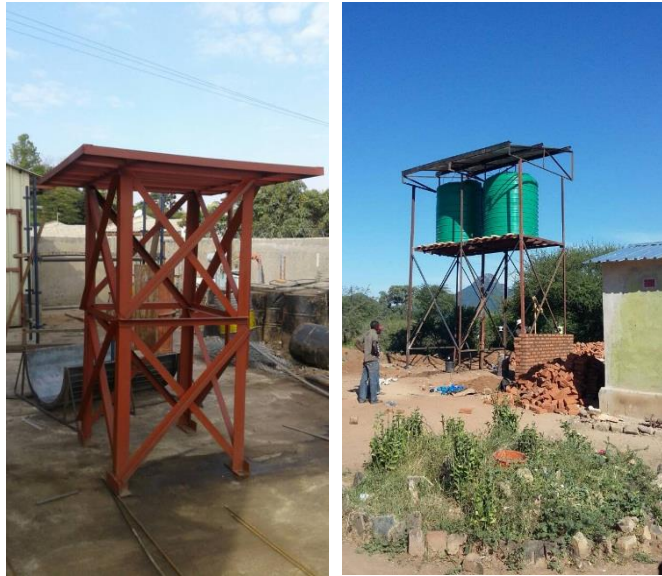
Figure 19 Fabrication of Mild steel Tank and Solar Support
