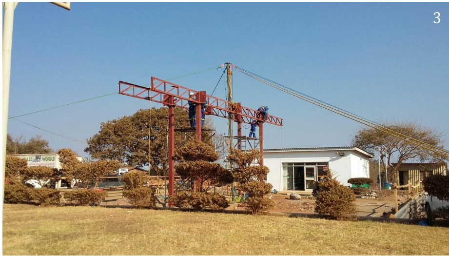
Figure 14 Above Fabrication and installation of Ntchisi Puma Filling Station
