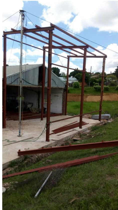
Figure 22 Fabrication and installation of Crate Crusher Shade at Carlsberg Malawi
