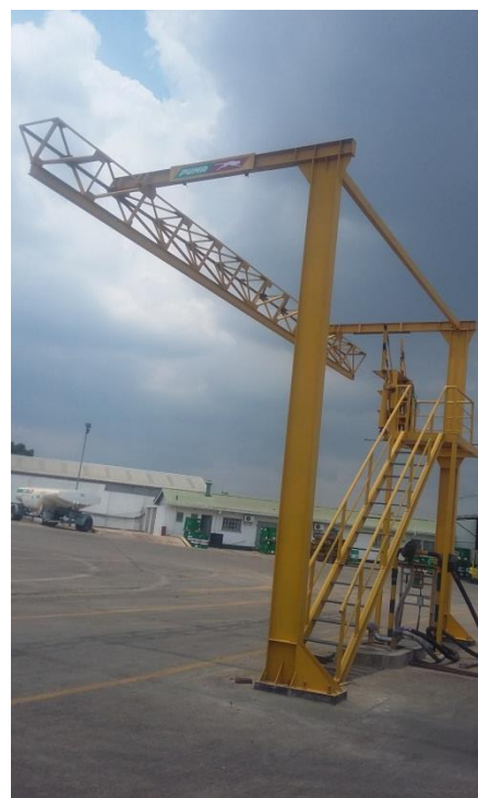
Figure 17 Fabrication and installation of Fall Arrestor at Puma Depot in Makata Blantyre
