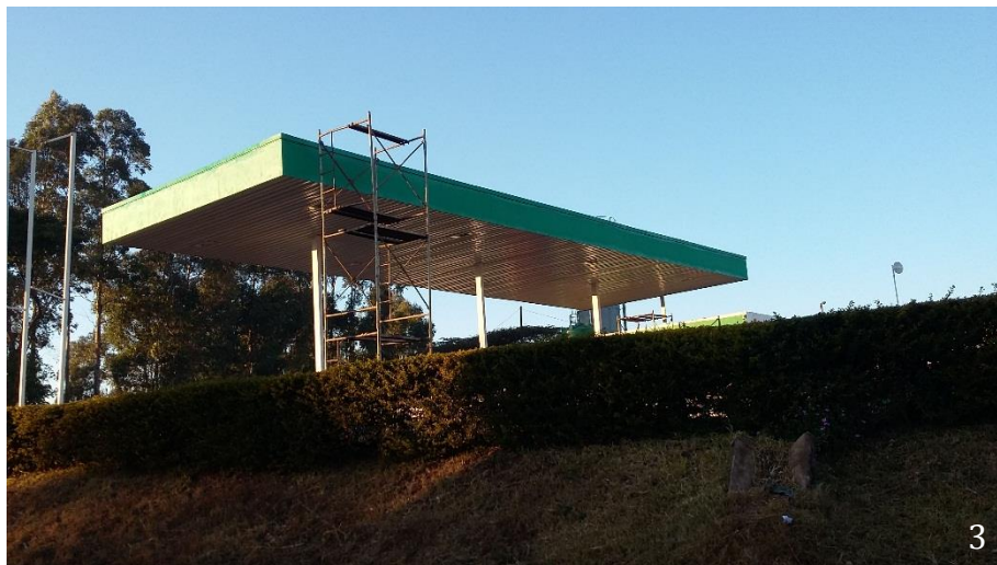
Figure 13 above Fabrication and Installation of Dedza Puma Filling Station
