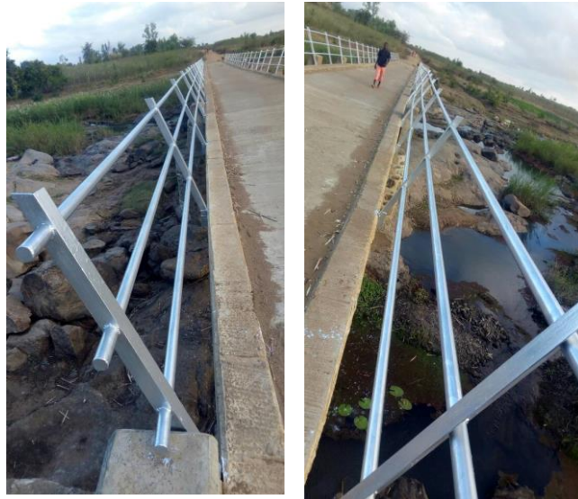
Figure 24 Fabrication and Installation of mild steel balustrades Thuchila bridge
