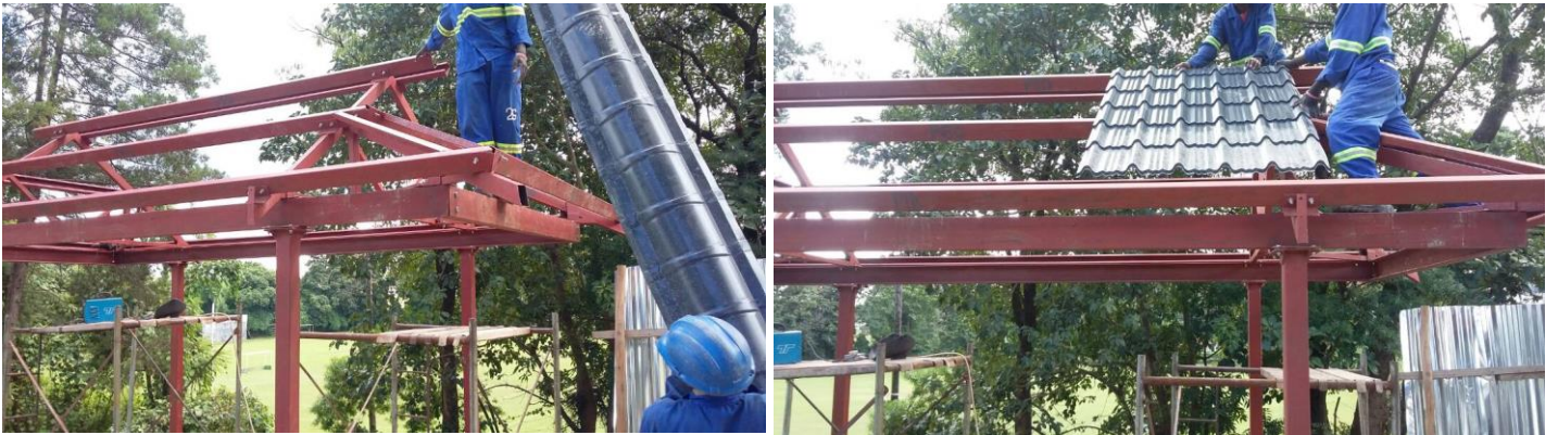
Figure 20 fabrication and installation of mild steel shed at Blantyre sports club
