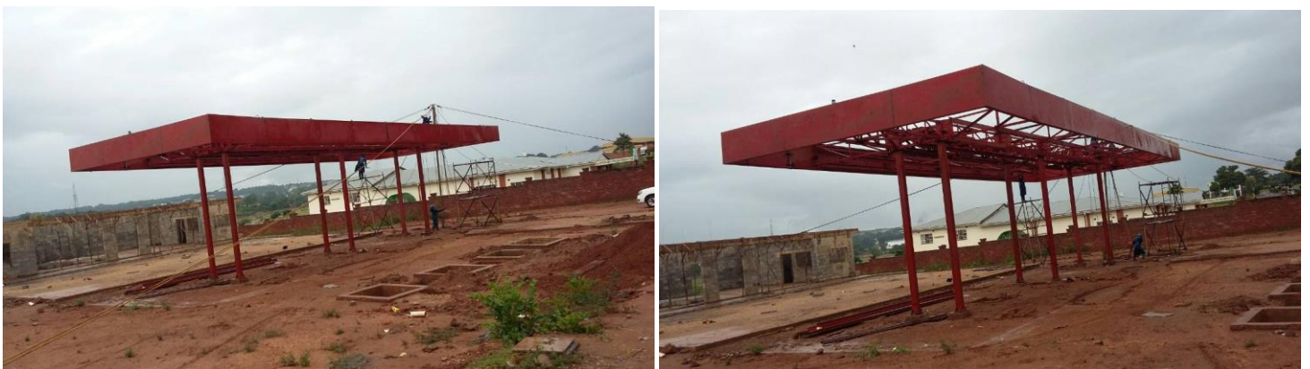
Figure 21 Fabrication of Lilongwe Area 2 Puma Filing Station
