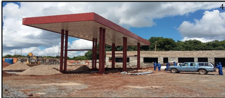
Figure 10 Above Fabrication and Installation of Bunda Turn off Total
